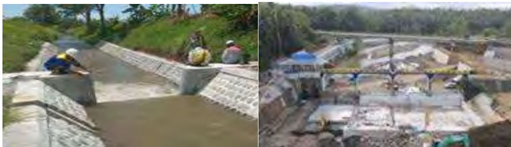
Figure 4. Left: Kedungputri Canals, Right: ME Gates at Weir (Serayu Opak RBO, 2023)
