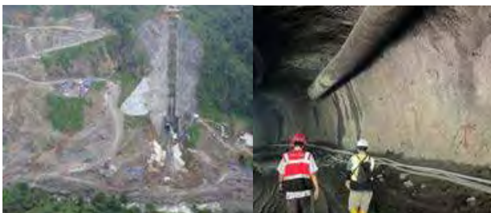
Figure 2. Bener Dam Progress July 2023 (Serayu Opak RBO, 2023)
