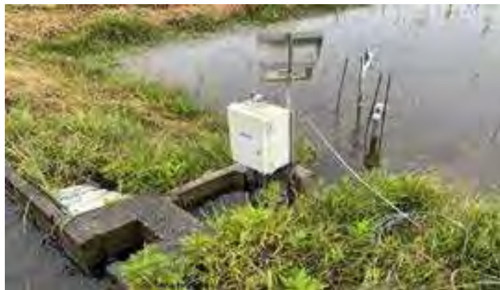
Figure 1. Paditch Gate (ICT smart automated sluice gate) installed at the observation plot.
