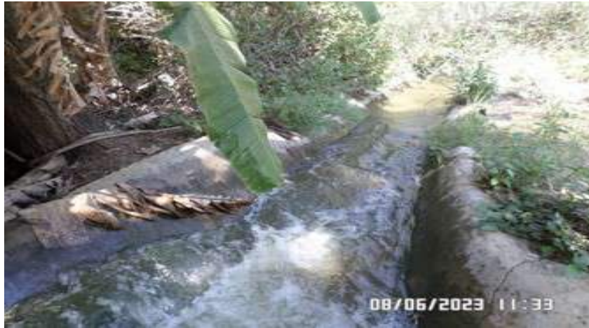
Figure 8: Drainage Canal Delivering Water to the Reservoir
