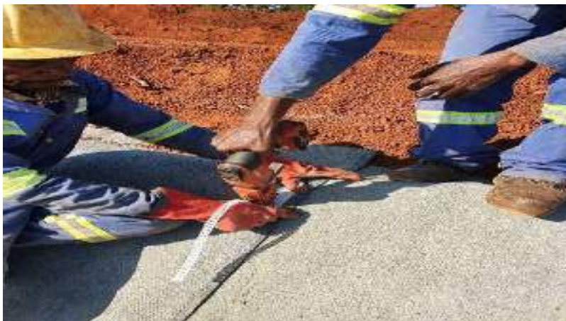
Figure 11. Screw fixing overlaps
