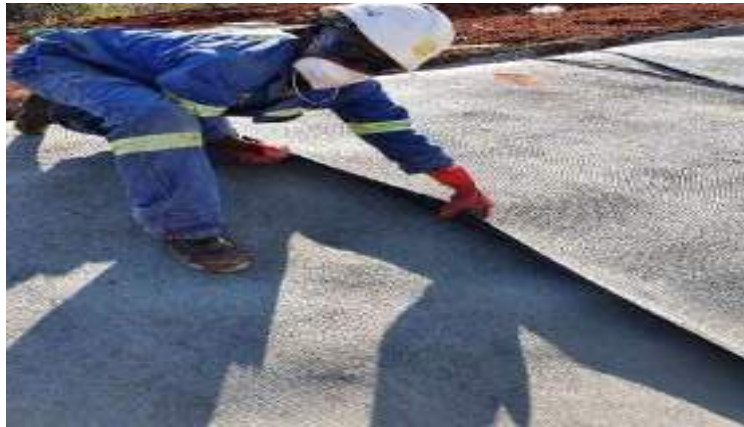
Figure 9. Cleaning GCCM backing
