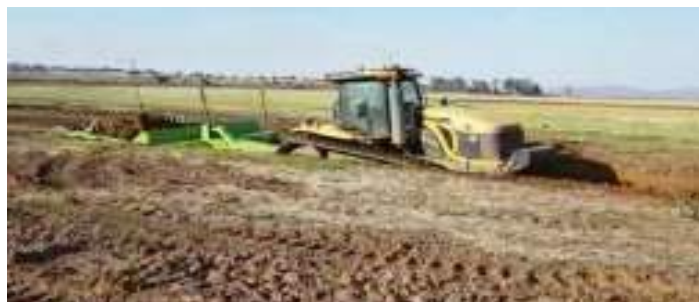
Figure 30: Construction of drainage Channel ( Source; Trevor Beaumont )
