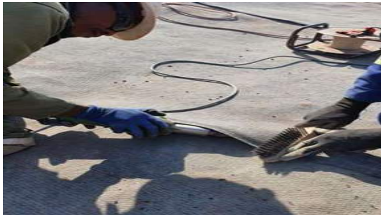
Figure 10. Thermally bonding overlaps
