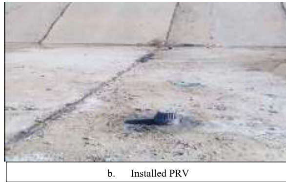
Figure 14. Installed PRVs at RD 110+200
