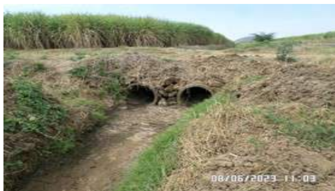
Figure 23: Asbestos Pipe Aqueducts
