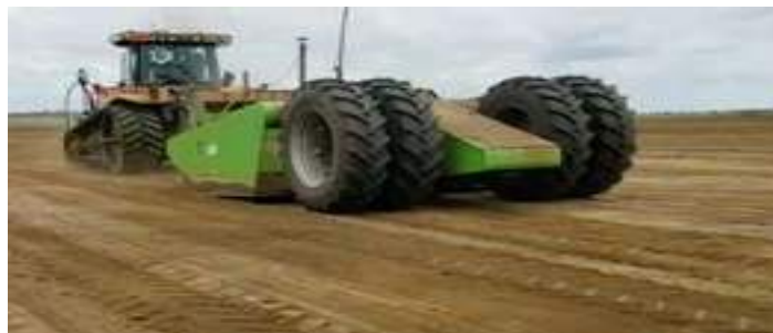
Figure 29: GPS guided cut fill scrapper
