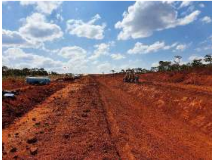
Figure 4. 8m wide canal profile preparation
