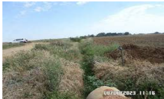
Figure 25: Concrete Pipe Culvert
