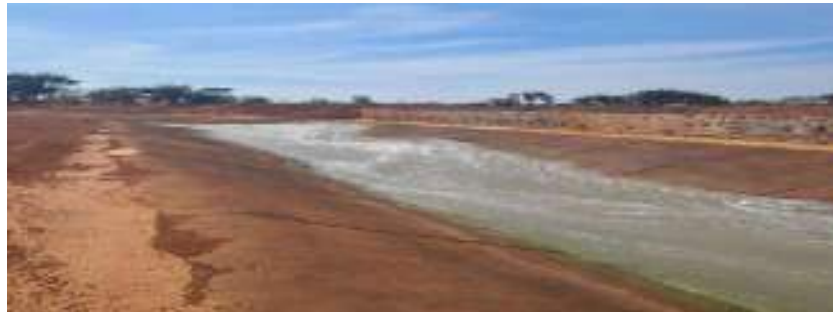
Figure 14. Drainage Canal in operation
