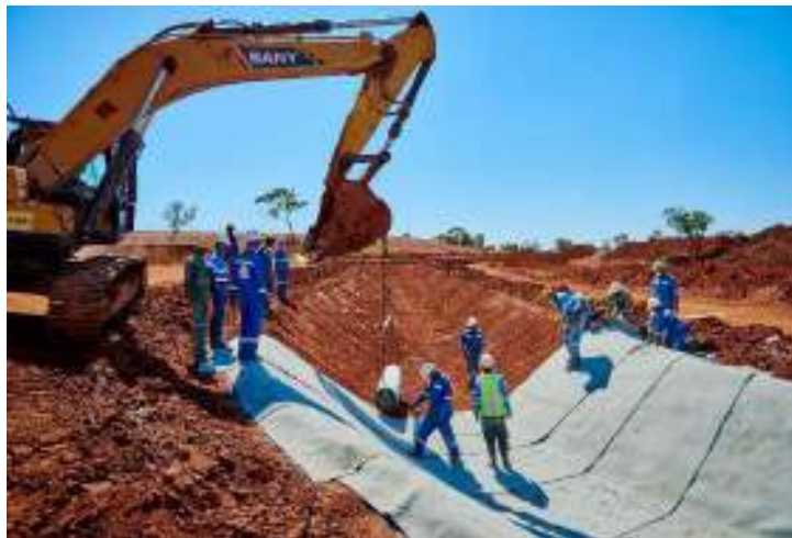
Figure 5. GCCM deployment from excavator deployed spreader beam
