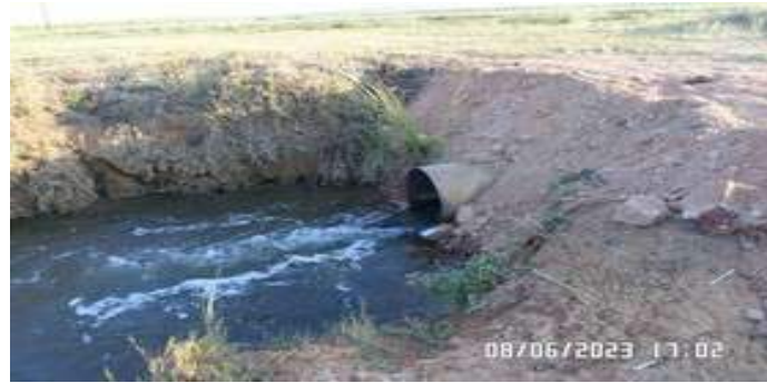
Figure 24: Steel pipe Aqueduct
