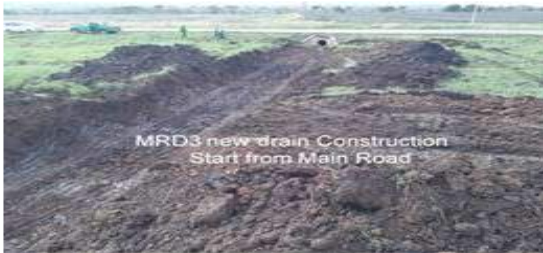
Figure 19: Construction of a Drainage Channel (Source: Trevor Beaumont)
