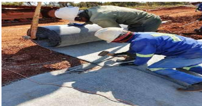
Figure 7. Inserting anchor pegs
