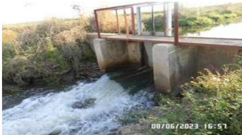
Figure 15: Sluice Gate Regulating Drainage Water reuse
