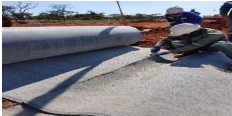
Figure 6. Cutting GCCM to length
