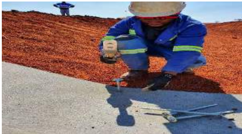
Figure 8. Inserting intermediate pegs
