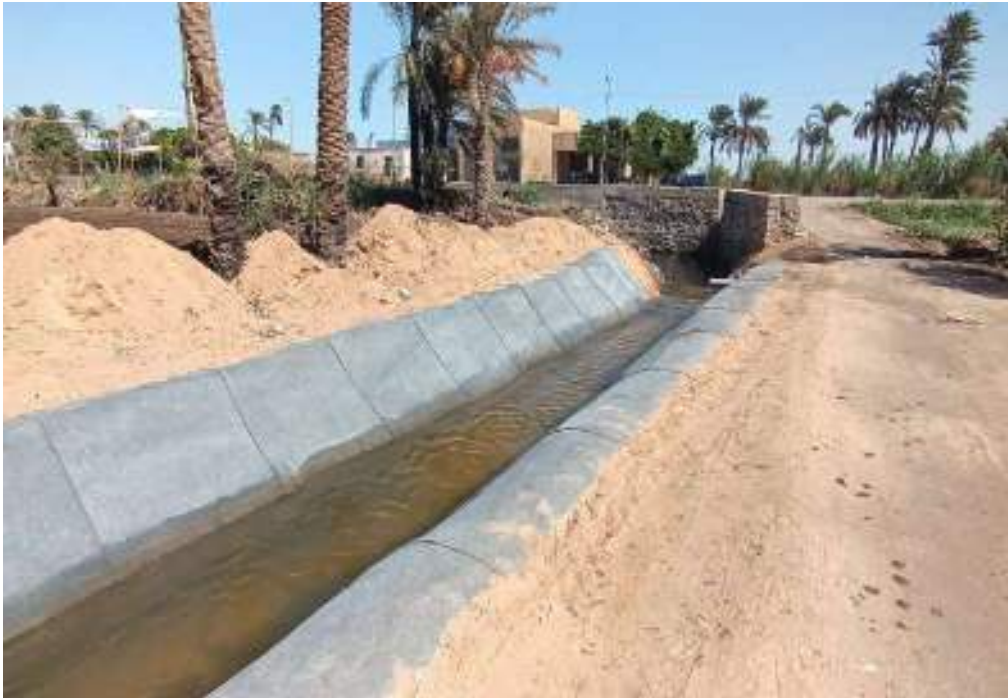
Fig 1. Atfih, Egypt Type II GCCM canal lining trial at completion
