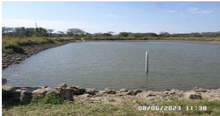
Figure 9: Reuse WATER Reservoir Storage
