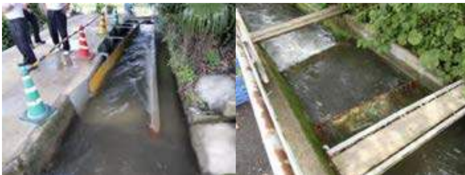
Figure 21 Aspect of channel near inlet
