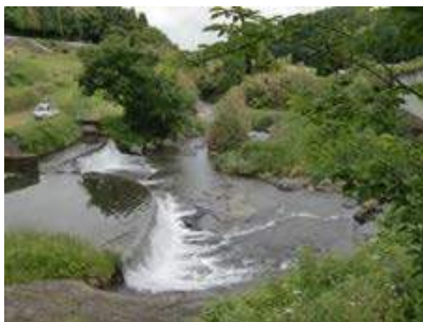
Figure 18 Kanda diversion weir at the source of the Kibaru-iro irrigation channel
