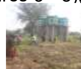
Figure 4: Tanks storing water pumped by solar to irrigate by micro irrigation.
