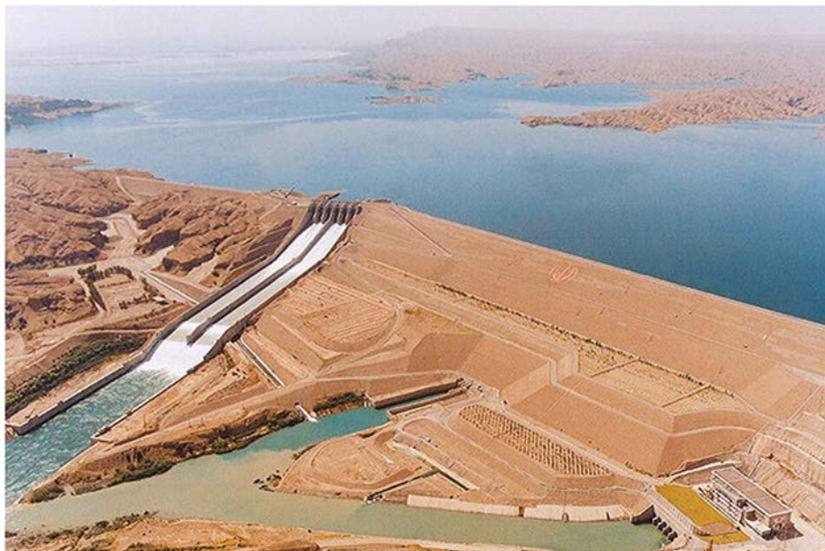
Figure 9. A general View of Karkheh Dam. [Colour figure can be viewed at wileyonlinelibrary.com ]
