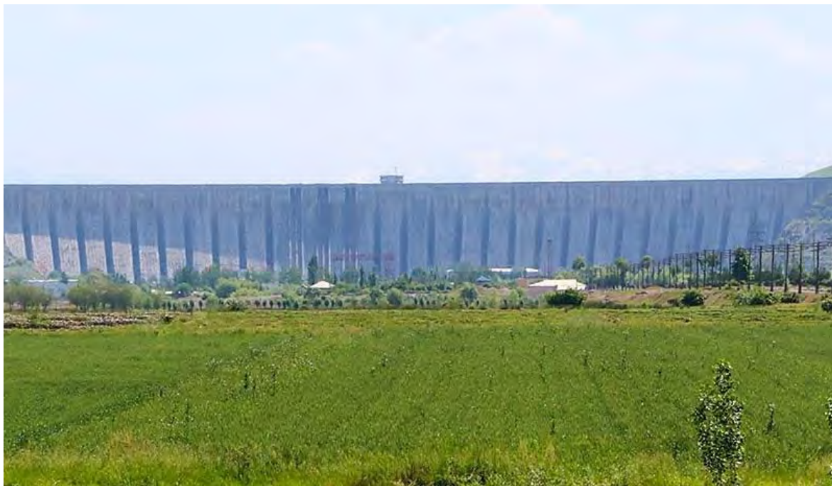
Figure 9. “Kampirravot” dam built on the Karadarya river. It was designed in 1962 and was completed in 1968-1982. The total length 1020 m. Dam is massive concrete with double buttresses-875 m. Maximum height 115 m.
