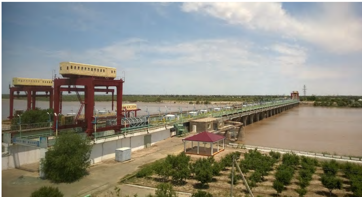
Figure 10. Takhiatash hydrostructure on the Amudarya river in Karakalpakstan (the biggest water weir in Central Asia completed in 1974) – capacity more than 11000 m 3 /sec
