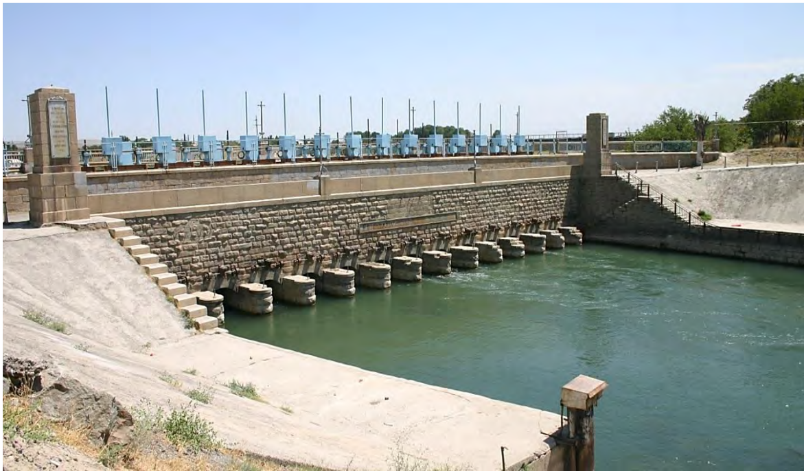
Figure 4. The head structure at the Dustlik (“Friendship”) canal (in the Soviet years, the Kirov Canal. It starts from the derivation channel of the Farhad hydroelectric station.
