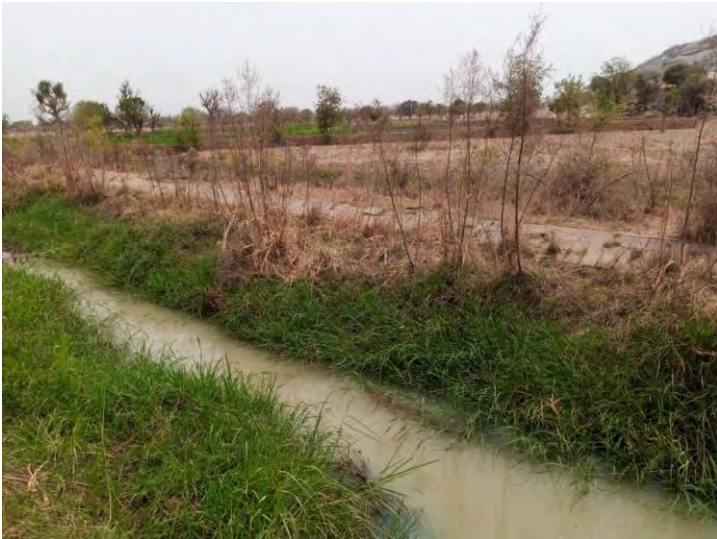
24km East Branch Canal- KRIS- Before
