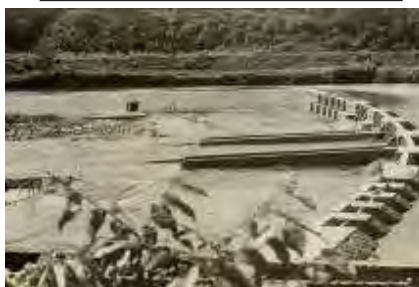
Previous Head Works made by the manufactured stone
