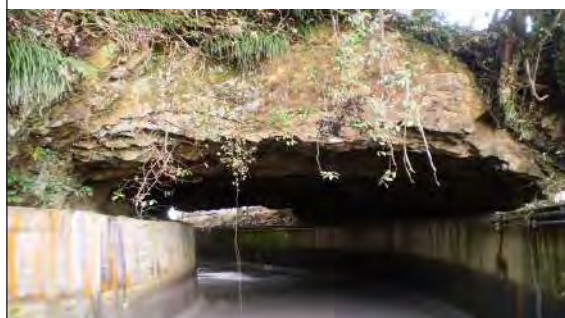
Remains of the original rock excavation work
