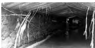
Former Iwasaki Tunnel
