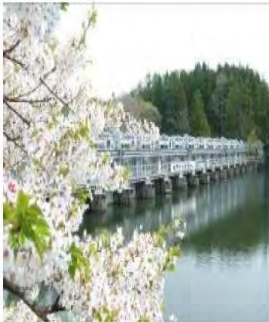
Jurokkyo Sluice (current photo)
