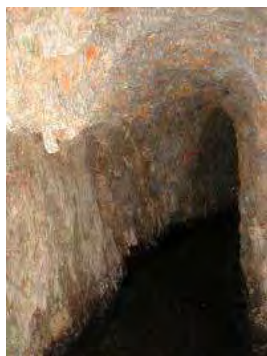
Tunnel at Teragaikae Waterway
