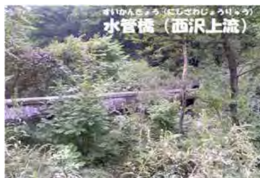
The aqueduct bridge
