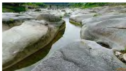
Canal remaining trace of rock excavation
