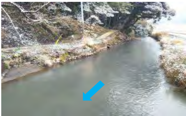
“Uwa-ide” irrigation canal The irrigation canal is paved. (1)
