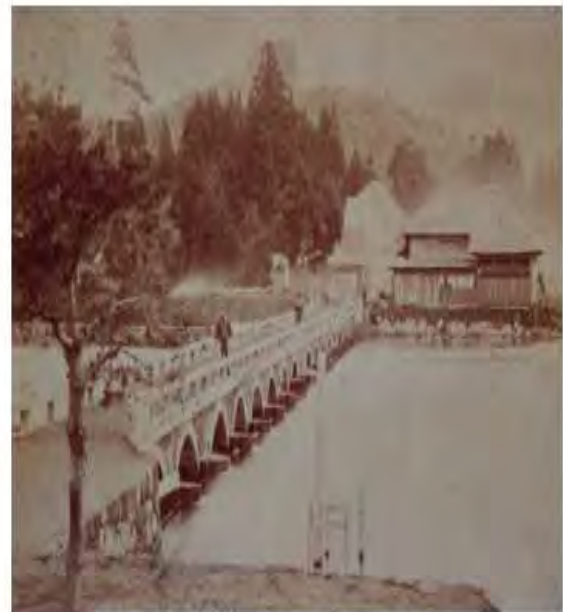
Jurokkyo Sluice (photo taken in 1882)
