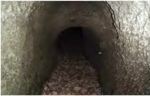
Tunnel was dug by man power using a chisel. It was dug from both sides and then joined. (Designated as Historic Site of Nagano Prefecture in 1981.)
