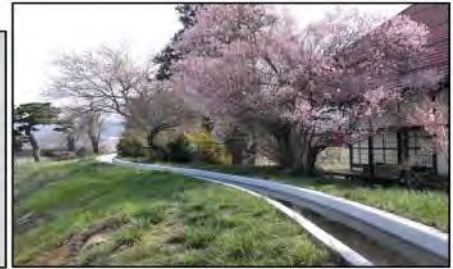
Tsukiseki Ground level of this section was low, so Gorobe constructed a high embankment and excavated a waterway through it.
