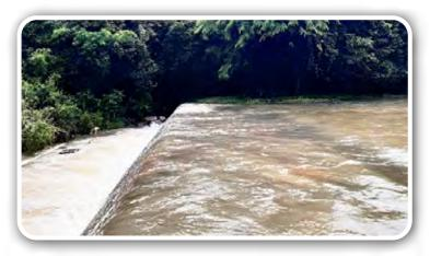
Ethimale tank is to be rehabilitated and augmented under the proposed Kumbukkan Oya reservoir project funded by GOSL. Identified major rehabilitation are such as raising of spill level, renovation of rip rap, strengthening of the dam, establishment of bathing steps, establishment of tor filter & toe drain, installation of piezometers on d/s slope of the dam, construction of access road for inspection, installation of levelling monuments and installation of boundary stones.
