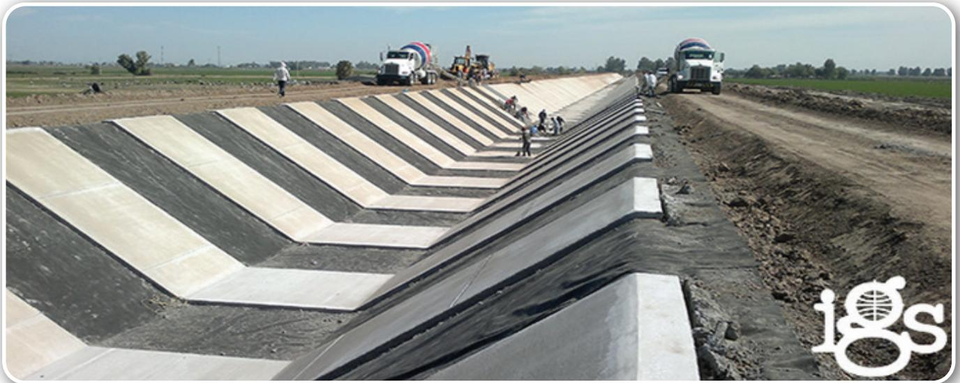
Geomembrane-lined canal in the process of being covered by concrete (credit: IGS Photo Competition, 2014)
