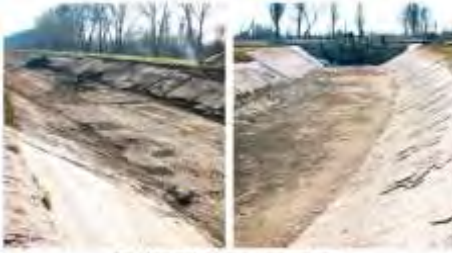
Figure 1.1. Perfect canal system. Reinforced concrete-lined canals.
